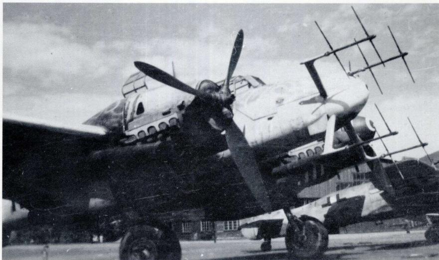
ABOVE AND ABOVE RIGHT: This abandoned Bf 110 G-4 was found by US forces at Bad Langensalza in April or May 1945. This particular machine, W.Nr. 110509, flown by 8./NJG 1, was coded G9+VS and lacked any radar aerials when photographed. On the starboard side, just visible protruding from the underside of the nose in the photograph (ABOVE) is the small plate which ensured that spent cartridge cases were deflected away from the propeller.
