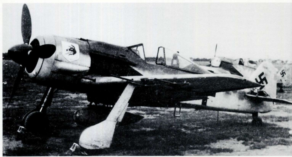
ABOVE, LEFT AND BELOW: Migge's Fw 190 A-8 'White 9' of 1./NJG 10 showing the acrials for the FuG 217 radar mounted on the starboard wing and the anti-glare shield over the exhaust. The badge on the cowlng originated with JG 300 and symbolised the unit's 'Wilde Sau' tactics. It appeared in various forms and was also used by NJGr 10. The photograph above shows the particular variation of the badge carried on the engine cowling of Migge's 'White 9'.
