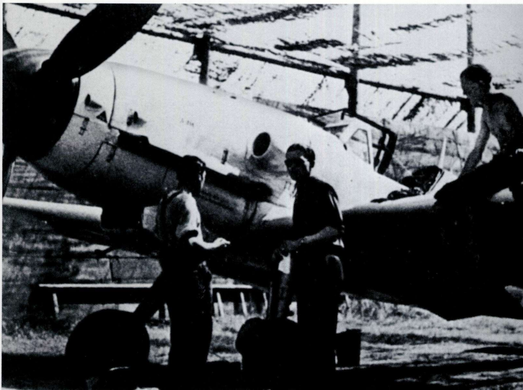
ABOVE: A late-production Bf 109 G-10 of I./NJG 11 at Bonn-Hangelar. This aircraft, 'White 11', was finished in a late war camouflage scheme of 81 and 82 on the uppersurfaces with 76 on the undersurfaces. Although not visible in the photograph, this aircraft had a long tail wheel and tall rudder.
