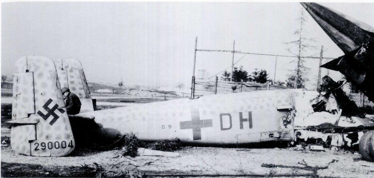
LEFT AND BELOW: This He 219, W.Nr. 290004, was found at Paderborn airfield on 10 April 1945 and was the first example of the type to be examined by the Allies. Although the nose, centre section and left wing were burned out, considerable information was obtained from an examination of the remains. Note that all the tactical code, G9+DH, was in black with the aircraft letter 'D' narrowly outlined in white.
