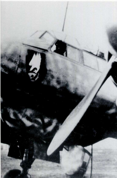
ABOVE: A Ju 88 C-6 night fighter of the 4. Staffel of an unidentified Nachtjagdgeschwader. The camouflage consists of 76 undersurfaces and plain 75 on the uppersurfaces which has been extended well down the fuselage sides. The 75 was then oversprayed with what appears to be 76 but in such a way that small patches of 75 remained. Such a finish, referred to in this work as 'reverse mottling', is often mistaken for 75 mottles applied over 76.
